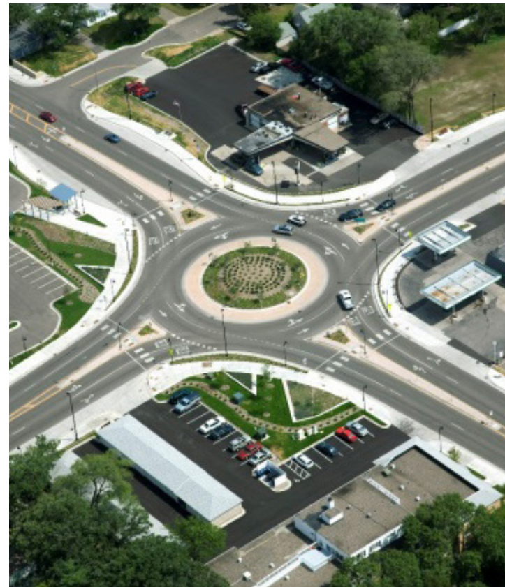
66th Street at Portland Avenue Roundabout Richfield, MN
