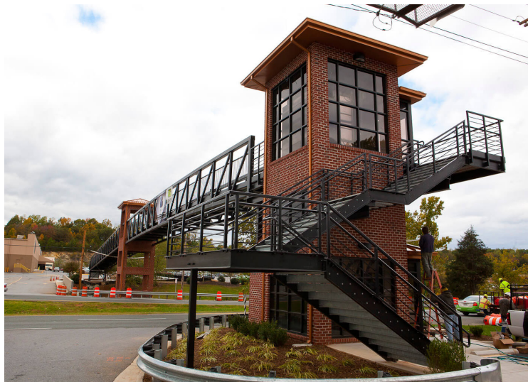
Wards Road Pedestrian Bridge Lynchburg, VA
