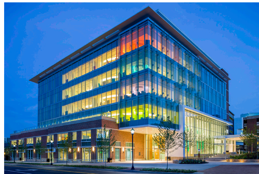
The Battle Building at the UVA Children's Hospital is LEED Certified Gold
