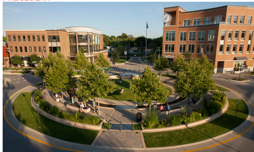
Roundabout with a Green Center Normal, IL
