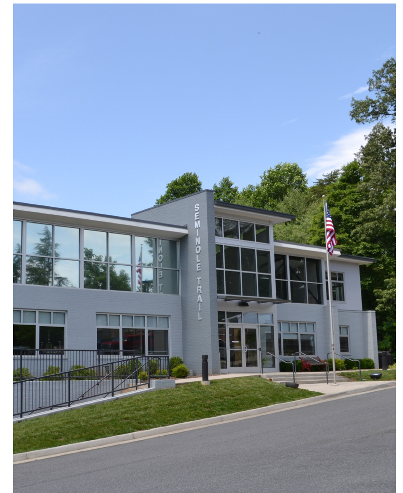
Seminole Trail Fire Station
