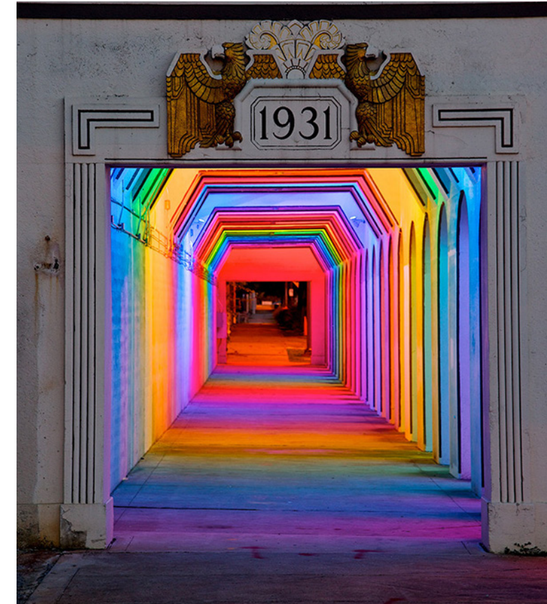
LightRails Pedestrian Underpass Birmingham, AL
