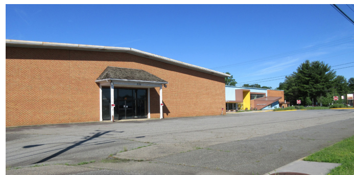
Vacant Warehouse Adjacent to Northside Library
